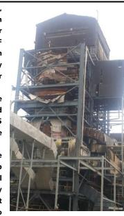
be in closed condition at panel. A momentary opening of fuel gas main valve by the operator to check the leakage in the flange resulted in formation of explosive mixture inside furnace of the boiler due to the passing valve. Operating procedure has been modified to prevent recurrence of this incident.
